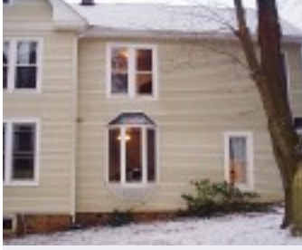
BEFORE: Tom and Kristen Chang wanted more space and a larger kitchen in their 100-year-old Victorian home. They hired John Broman, an aerospace engineer, to build their two-story addition.
